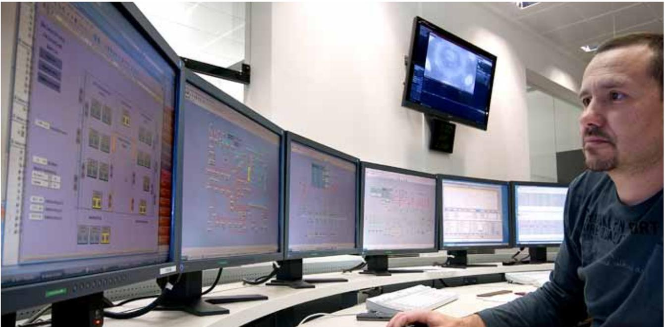
*All eight workspaces in the areas of medium-voltage (six workspaces) and high-voltage (two workspaces) are each equipped with six monitors and thus ensure an optimum overview of all data and processes. User-friendliness is also considered: all six monitors can be operated with a single mouse, which also increases working efficiency considerably.*
